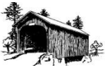
Maine's oldest covered bridge was built in 1840. It spans the Presumpscot river.
